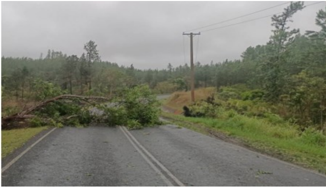
Figure 13e: Nawau, Queens Road. Source: Fiji Roads Authority.
