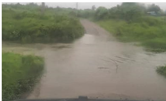
Figure 12b: Vatuwaqa Crossing, Sereva on the 13 th November. Source: National Disaster Management Office
