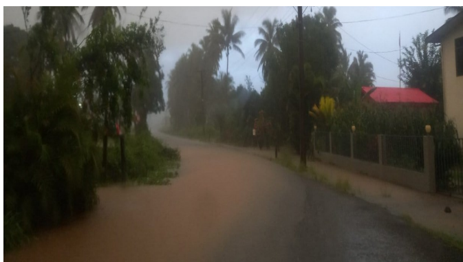
Figure 12i: Vakabalea Road in Navua on the 28 th November. Source: Fiji Roads Authority
