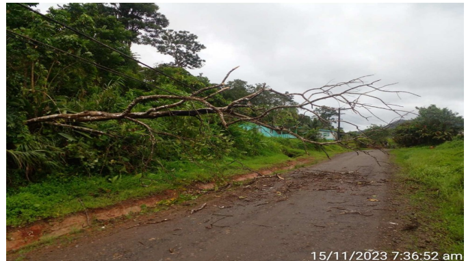
Figure 13h: Nabukaluka Delailasakau Road, Central Division. Source: Fiji Roads Authority.
