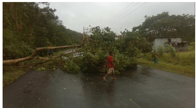
Figure 13l: Kings road Rakiraki near Rokovuaka. Source: Fiji Roads Authority.
